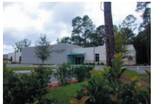
The Charles M. Neviasser Educational Institute, a 10,000 SF instructional facility in Jacksonville. This extension of the Community Hospice campus contains the Hospice Foundation for Caring, an education and outreach program, grief and bereavement services, and a venue for conducting research and development. TTV Architects, Inc. was in charge of the Schematic Design, Design Development, Construction Documents, and Construction Administration.
