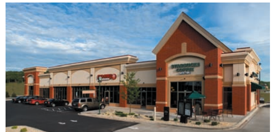
Ban Tara Development - The Ban Tara Lot Building sets the design precedent for future buildings in this new 22-acre retail development in a high visibility and high traffic count area. The building owners wanted to create a striking building that would draw customers. The 10,000 sq ft single-story building has a clear-span interior allowing flexibility for up to seven tenants.
