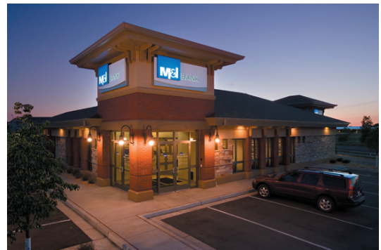
M&I Bank - This M&I Bank branch followed corporate prototypes for the interior, while creating a unique classic design for the exterior. The building features a prominent entrance tower, a tower over the three drive through lanes, and extensive brick, EIFS, and stone. Through creative site layout, Frisbie Architects was able to fit this bank with its 4,016 sq ft footprint on a small one-half acre site and have it meet all codes while functioning well.
