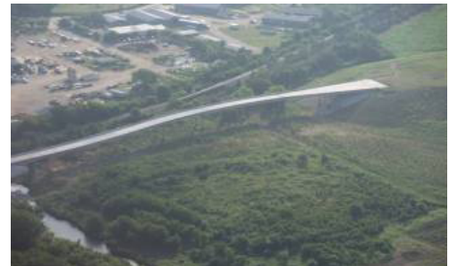
Salt Road Bridge, Fort Worth, Texas. A 1,431 foot long bridge for the City of Fort Worth, Texas to access their landfill.
